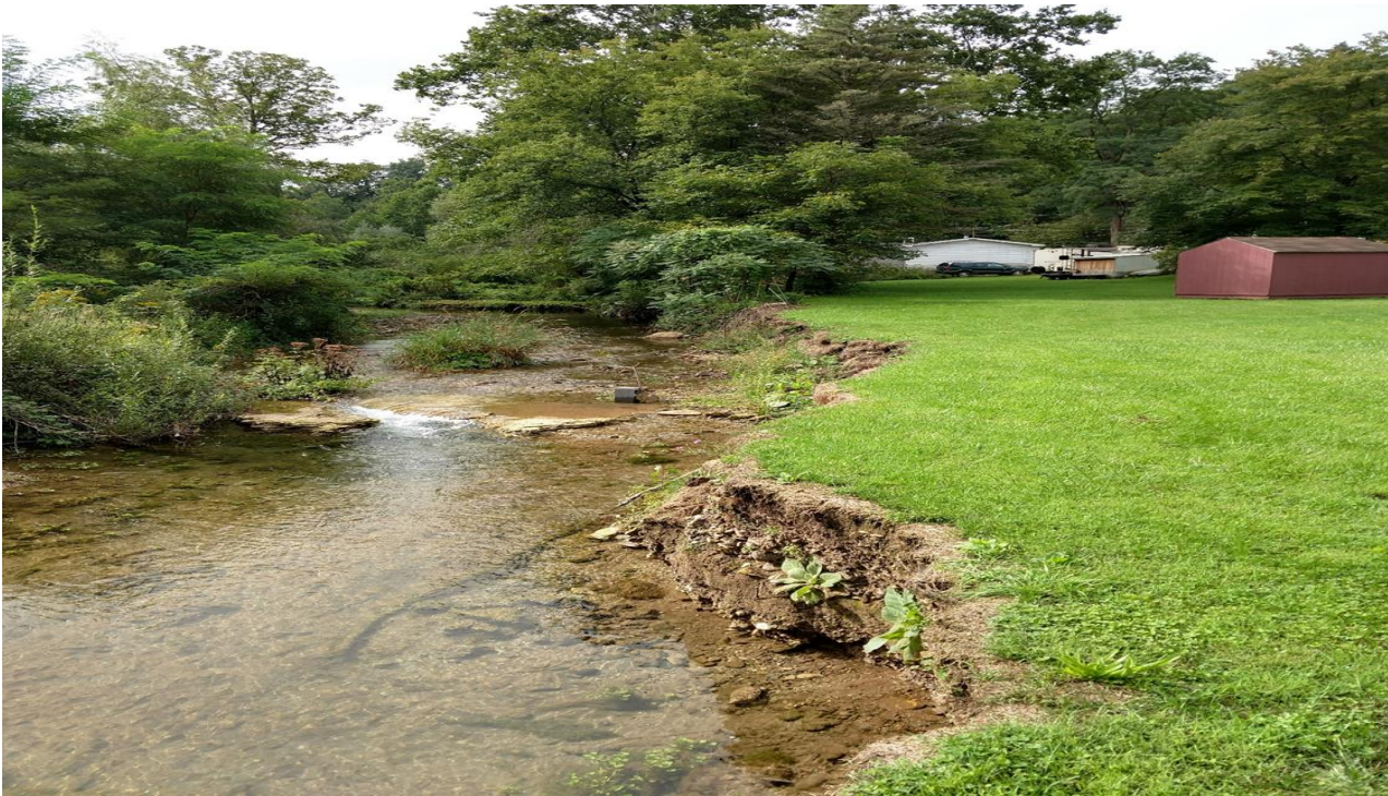
Severe erosion along a section of Canaseraga Creek was contributing significant amounts of sediment into the watershed. Project cost $24,000 – County, SWCD and Landowner.
