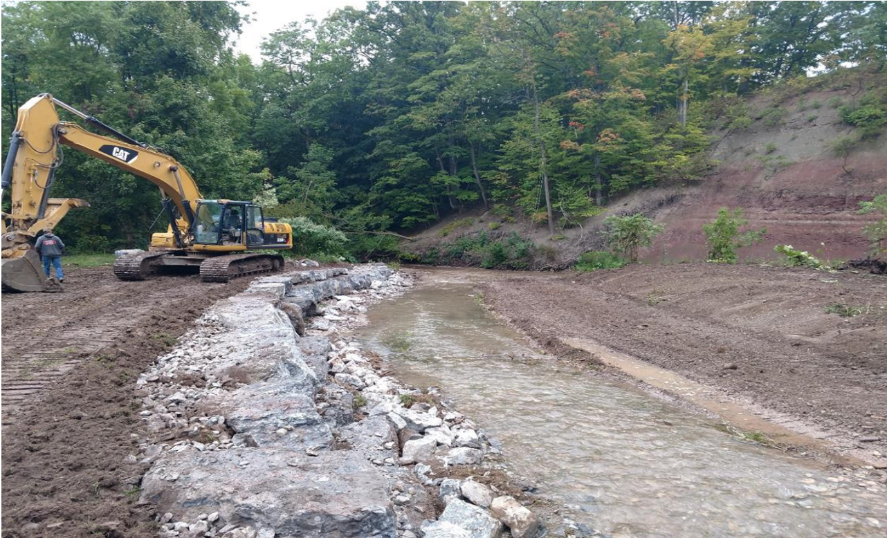
Structural stabilization and reconnecting the stream to the flood plain will dramatically reduce the amount of sediment coming from this location. Photo just prior to seeding and mulching of site.
