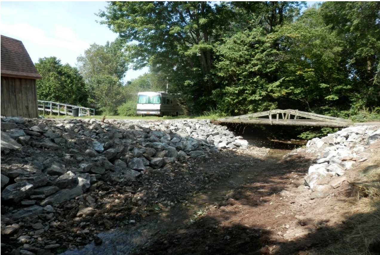
Streambank after structural stabilization to reduce erosion.
