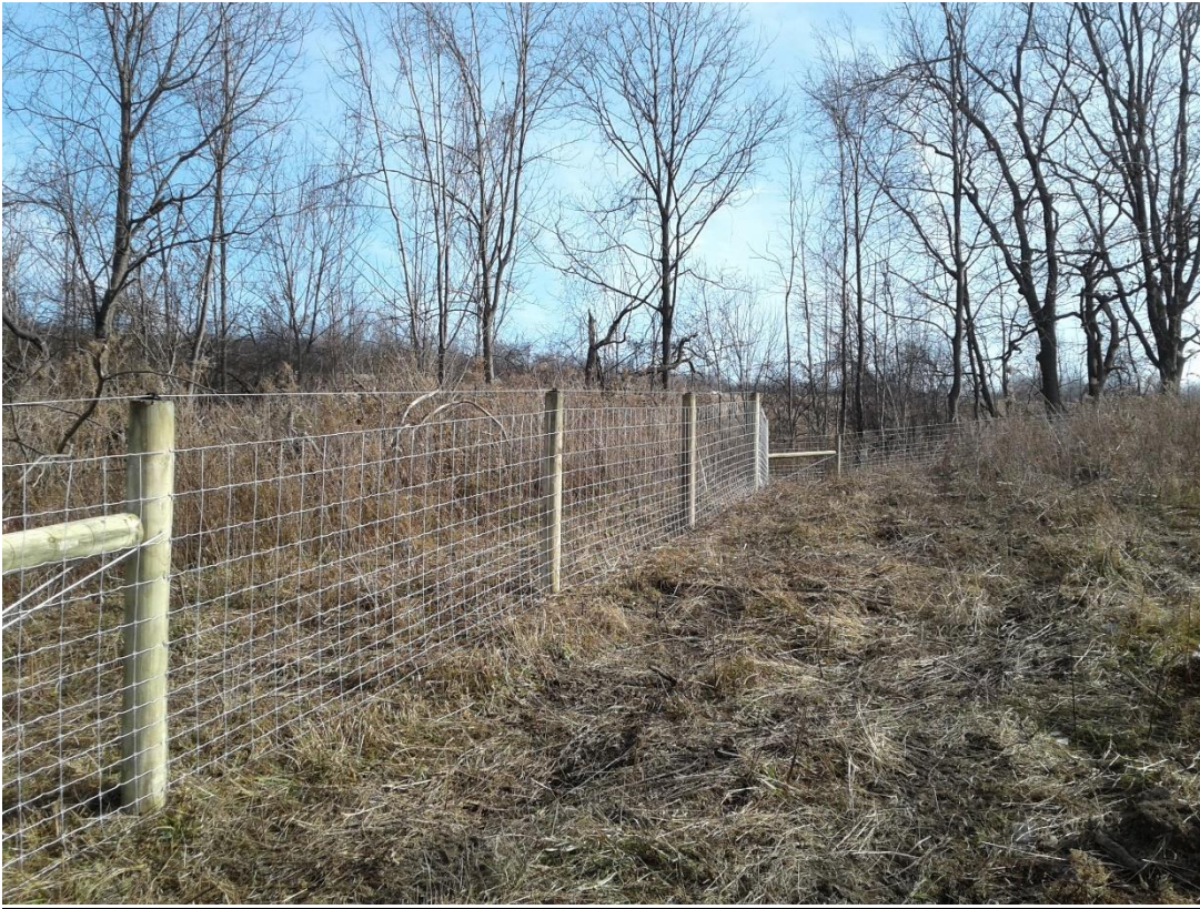
Woven wire perimeter fence installed as part of an 84-acre rotational grazing system on a sheep farm. Cost: $39,037. Source: NYS Environmental Protection Fund
