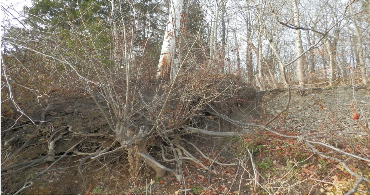
Erieville Reservoir bank protection (before implementation). Note the severe erosion.
