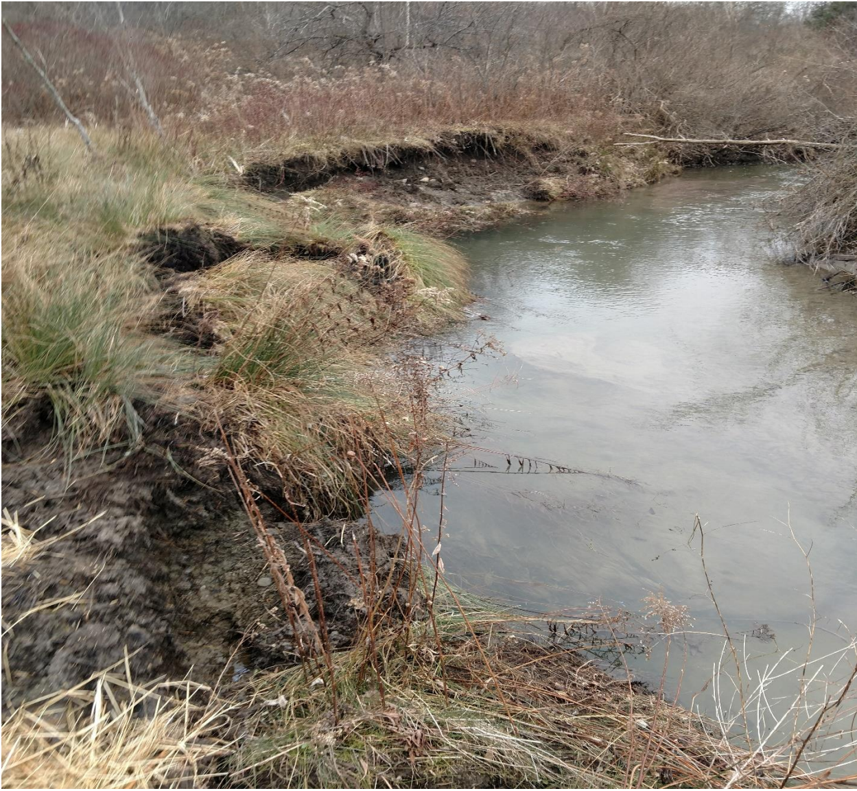
Severe erosion along Limestone creek is resulting in large quantities of sediment entering the stream.
