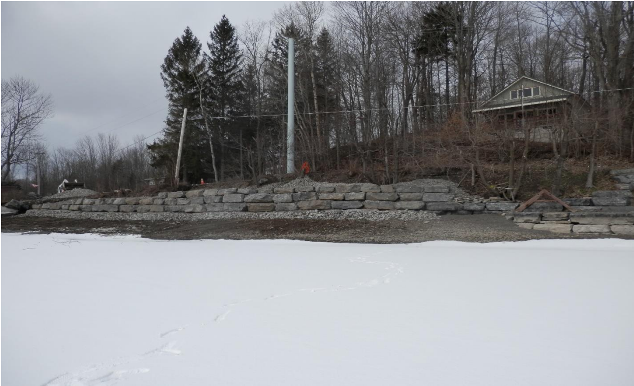
Reservoir bank after structural stabilization. – Cost $39,250 Funding - Madison County and Town of Nelson.
