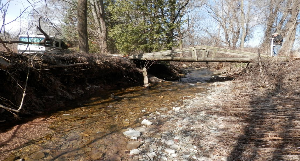
Severe erosion along a tributary to Oneida creek was contributing large volumes of sediment to the stream. Cost - $5,700 - County, Landowner.
